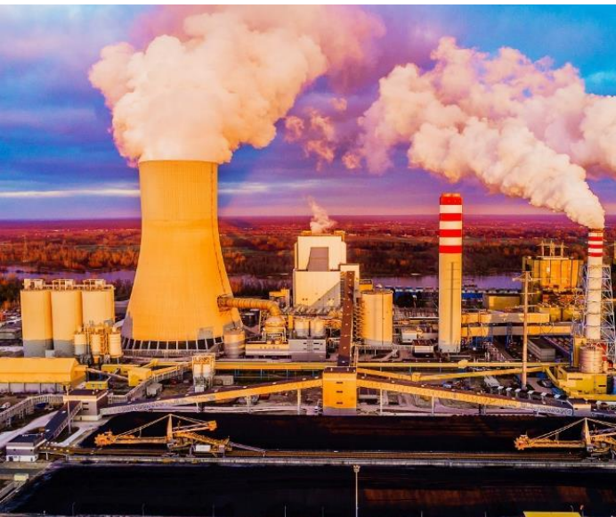
Unit B11 in Elektrowni Kozienice Power Plant
