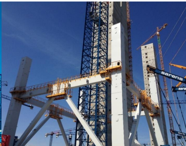
Truss structures, frames, poles
