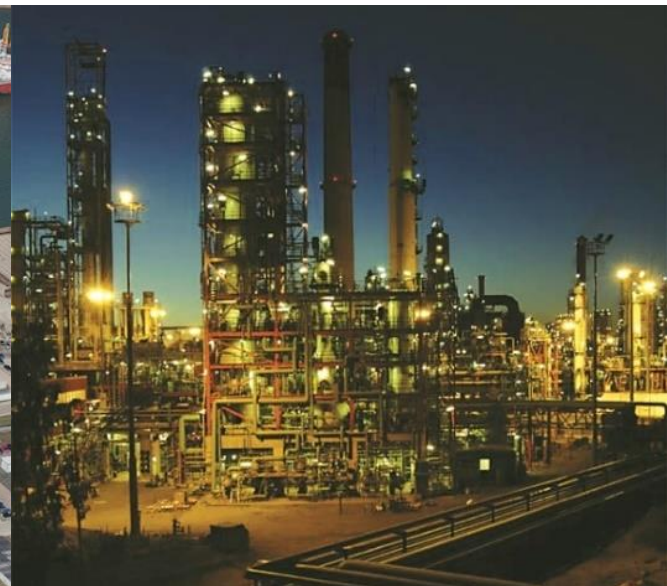
Biodiesel Installation for Porvoo, Finland
