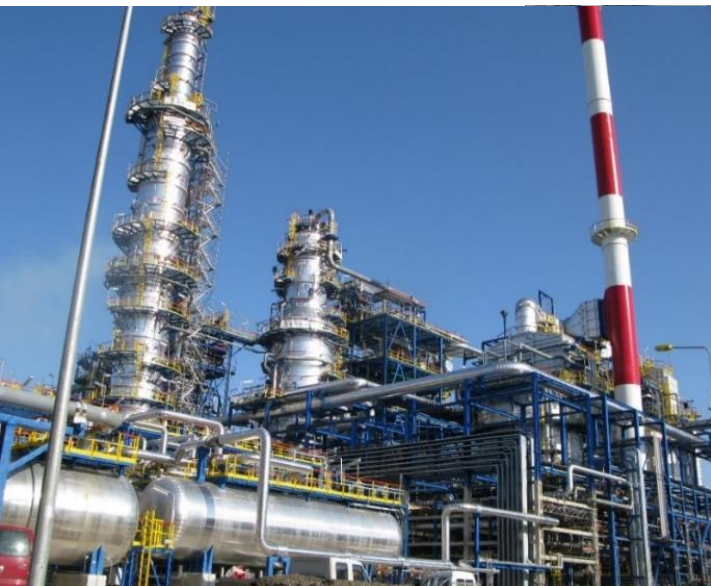
Construction of CDU/VDU installations Lotos Group Refinery in Gdańsk
