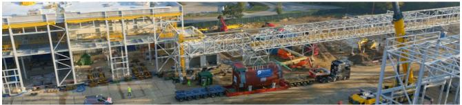
The foundation of the steam turbine at the construction site of the New Czechnica Combined Heat and Power Plant is ready. Installation of the first pieces of process equipment including the four peaking and reserve boilers begins. The construction of a gas-fired combined heat and power plant in Siechnice near Wrocław is a priority investment by Zespół Elektrociepłowni Wrocławskich KOGENERACJA S.A., part of the PGE Energia Ciepła Group.
